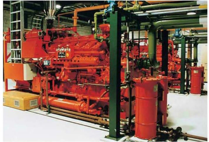
Figure 1-14. One typical application of stationary diesel engines. While these engines are permanently fixed, smaller diesel engines are transportable to any place where a powerful, efficient engine is needed.
